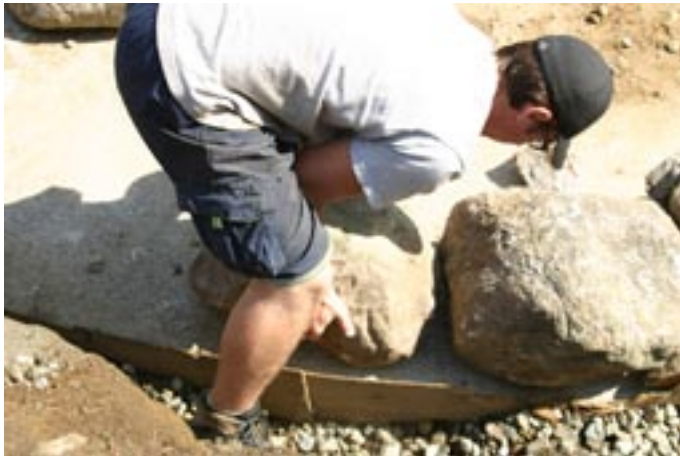
Field Stone Masonry
